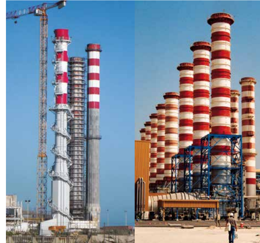
EXHAUST CHIMNEY BY PASS SYSTEM - GT ALSTOM
