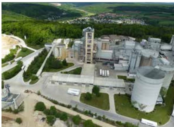
Figure 2. A high-dust SCR plant in the Solnhofen cement plant after recently conducted modifications. Source: Solnhofer Portland-Zementwerke.
