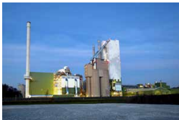
Figure 4. New IKN precalciner kiln in the Burglengenfeld plant in southern Germany Source: HeidelbergCement.
