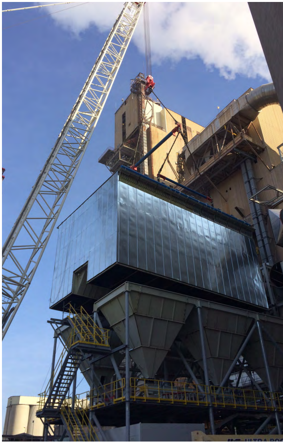
Boldrocchi's previous experience with a 'big lift', such as this one weighing 135 metric t, helped considerably.
