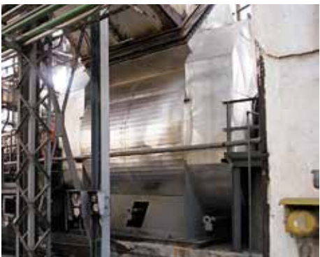
ID FAN WITH STEAM TURBINE
