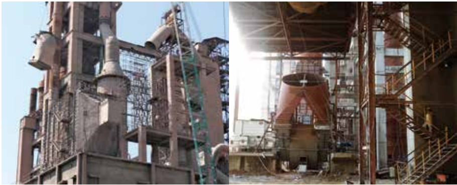
ESP TO BAG FILTER KILN ID FAN
