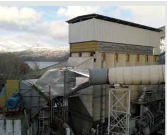
CONVERSION OF ESP IN BAG FILTER
